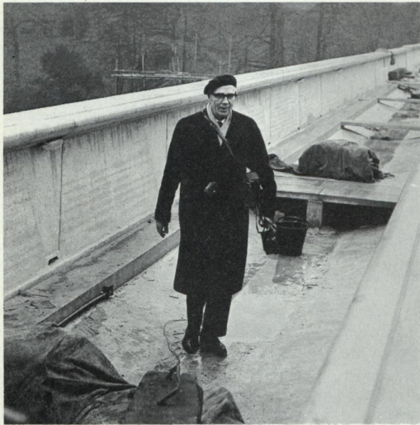
Ove Arup on the Kingsgate footbridge, Durham.
